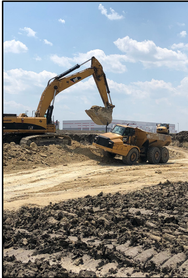
Workers excavate a site at Urban Mining Company's facility for manufacturing neodymium/iron/boron magnets in San Marcos, Texas.
